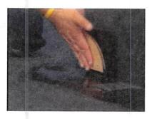
**Step 8**- Starting from the center; mold each side of the flashing around the corner.
