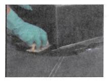
**Step 2**- Using a scrubber pad and holder; apply QuickPrime™ Plus Primer to a 14.0″ by 14.0″ (35.56 cm x 35.56 cm) area of the corner.
