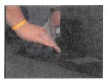
**Step 10-** Place your hands on the flashing, pushing down until the flashing extends 1.00" (2.54 cm) onto the horizontal surface and tightly into the 90° break.
