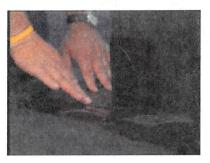
**Step 11-** Place your hands and fingers on the transition from the horizontal to the vertical. Mold the flashing into the transition by working from the vertical corner line out, in both directions and along the transition to the edges of the flashing.
