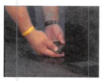
**Step 7**- Center the folded corner flashing against the corner edge with the short side facing the corner edge.
