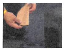
**Step 4**- Fold the corner flashing in half with the perforated edge on the bottom.
