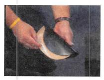
**Step 6**- Place the removed portion of the release paper in the folded flashing to facilitate installation.
